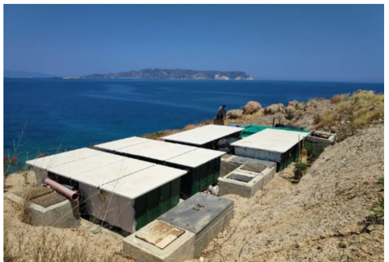
Cliff installation with no odours and noise.
