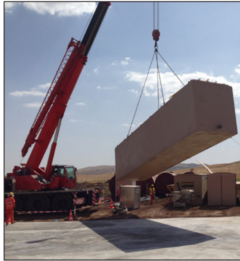
AX-Mobile units are completely pre-packaged and built inside a durable, insulated fiberglass tank that is easy to ship and set.
