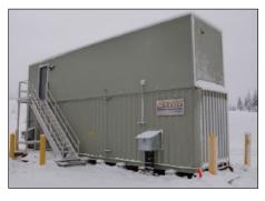
had to meet strict NPDES permit requirements for surface discharge, since subsurface discharge was not an option. The system was commissioned in December 2009 and sampling shows that effluent quality is averaging BOD of 6 mg/L, TSS of 5 mg/L, and 5.9 MPN/100 fecal coliform.
