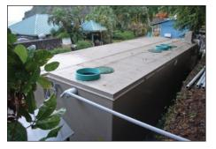
opening date. At only 7' (2.1 m) wide and 12,000 pounds (5443 kg), the units were trucked to the site, down steep narrow roads, on the back of a standard flatbed and lifted with a crane. Less than two days after reaching the site, the system was up and running, in spite of power fluctuations and other problems. This system includes a UV disinfection unit, and effluent sampling shows it is producing 7 mg/L BOD.
