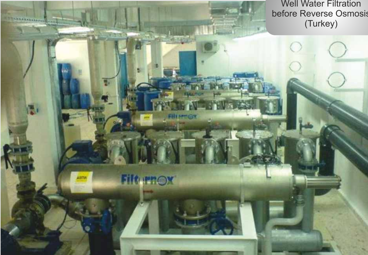
Replacing Sand Filters with Filternox ® Filters before Softeners (Turkey)
