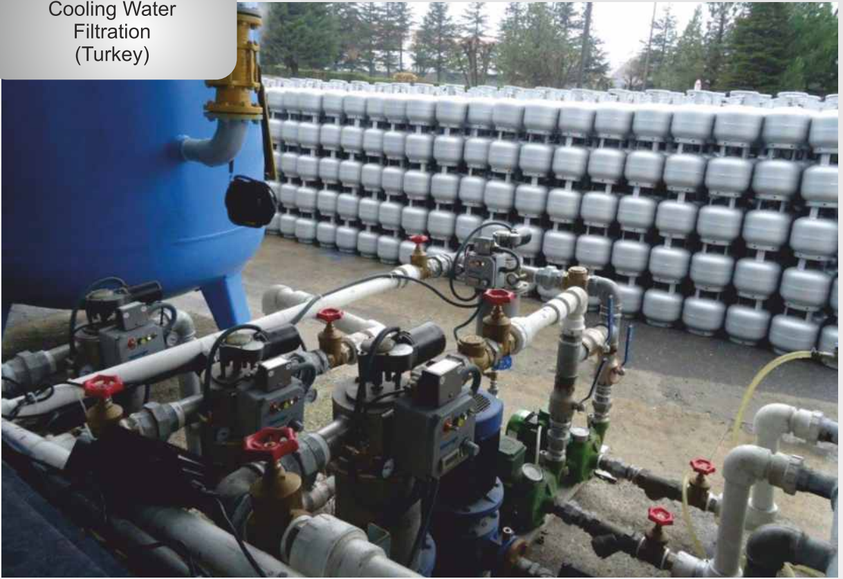
Plastic Industry Cooling Water Filtration (Turkey)
