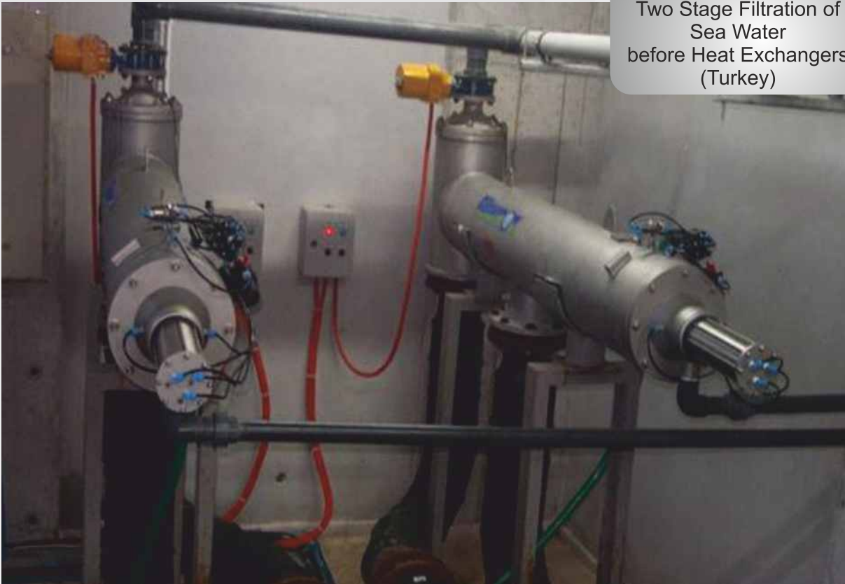
Two Stage Filtration of Sea Water before Heat Exchangers (Turkey)
