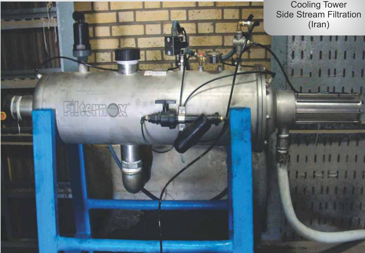
Cooling Water Filtration (Iran)
