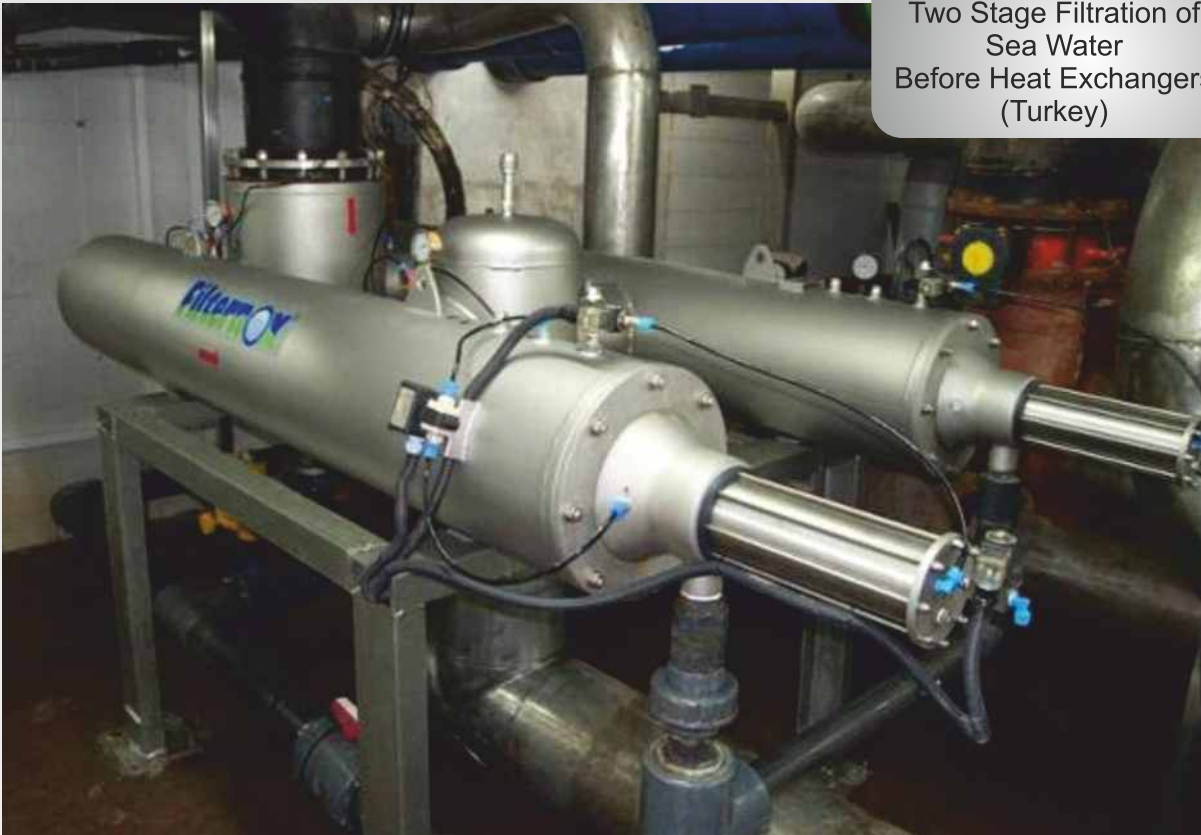
Two Stage Filtration of Sea Water Before Reverse Osmosis and Desalination (Turkey)
