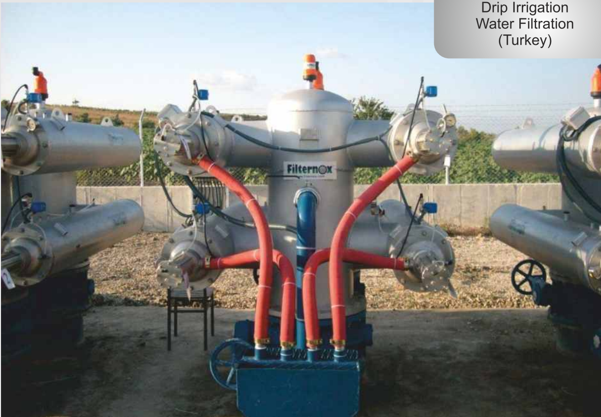
Drip Irrigation Water Filtration (Turkey)
