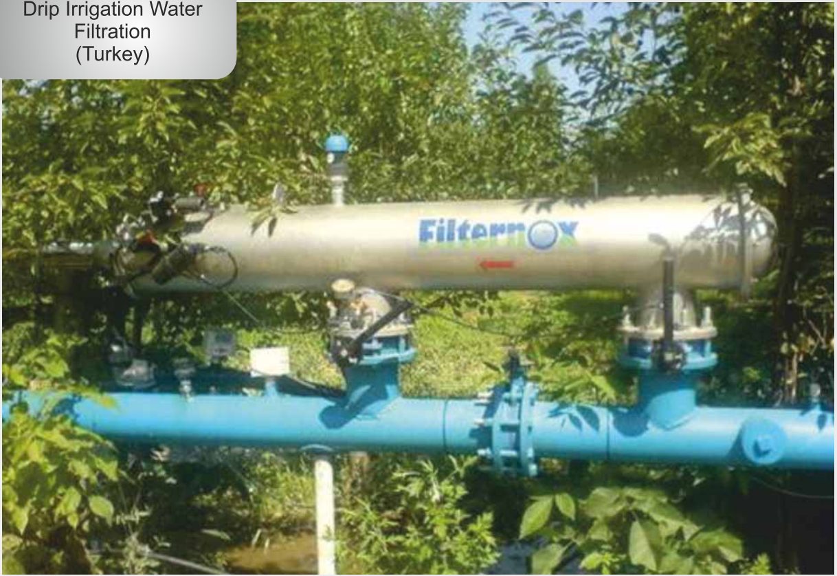
Drip Irrigation Water Filtration (Turkey)
