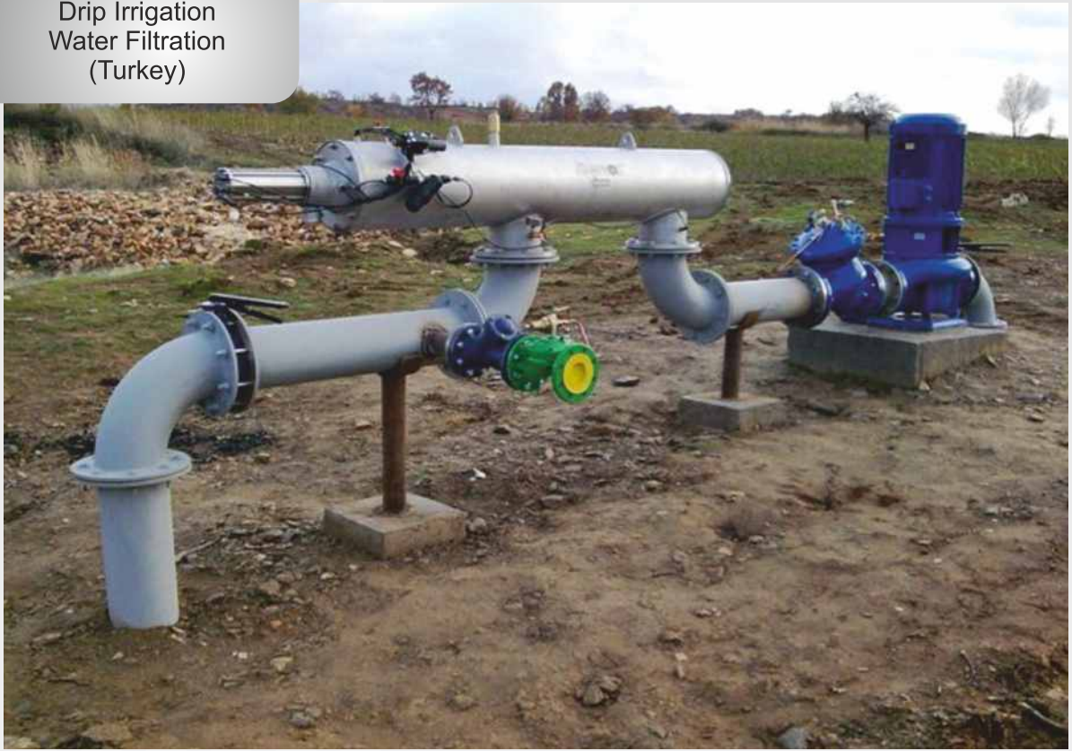
Drip Irrigation Water Filtration (Turkey)
